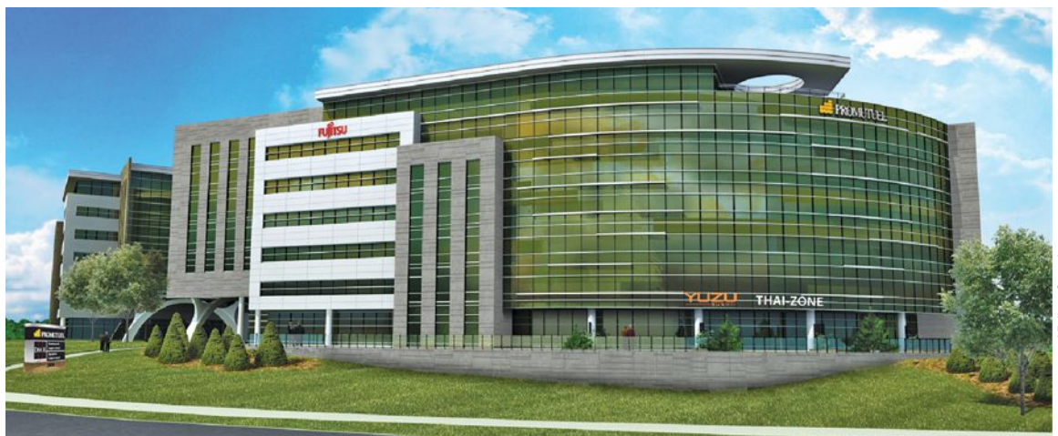
The Fujitsu Innovation Center represents a $20-million investment in Fujitsu's Québec City operation. The Center provides collaborative space where business partners and customers are invited to work with Fujitsu specialists to put new ideas into practice and build innovative business solutions.
